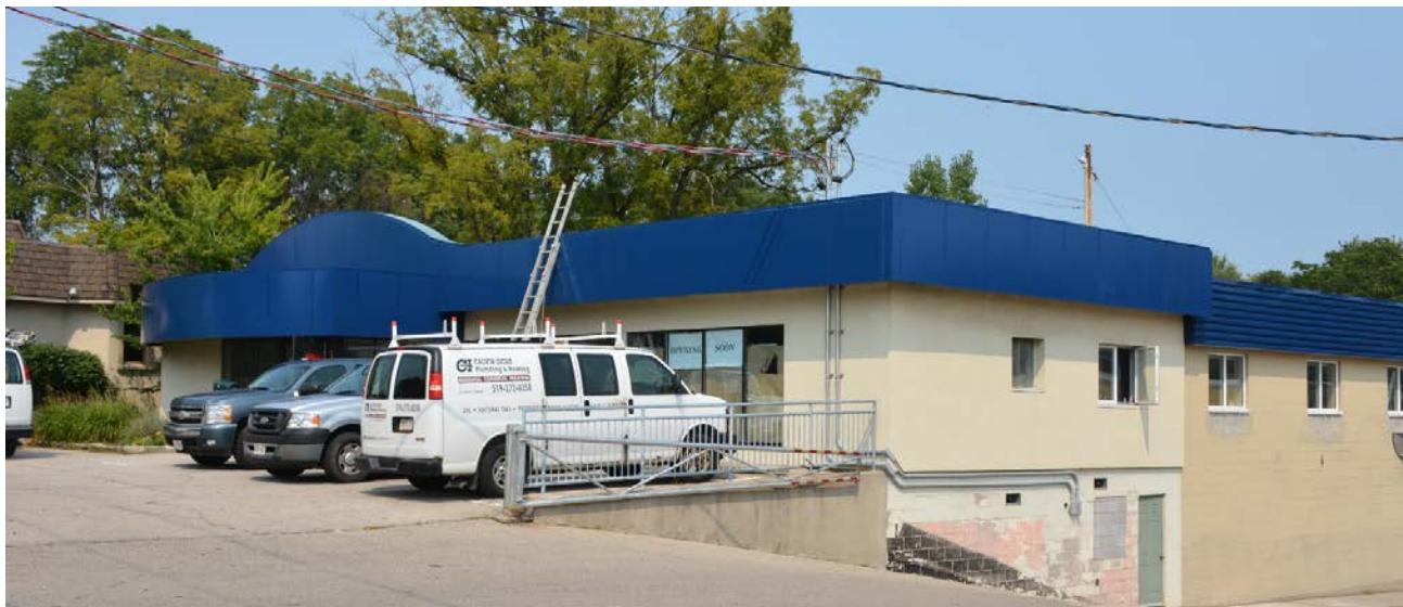
Picture 11 - Building Front/Side
