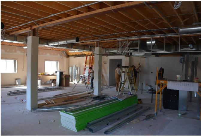
This picture (taken Sept 24<sup>th</sup>) shows bulkheads being installed for HVAC ducts. This has now been completed and drywalled in. Flooring has been delivered and ready for installation once painting has been completed. Millwork for the Bars is being done off-site and will be installed after the flooring.
